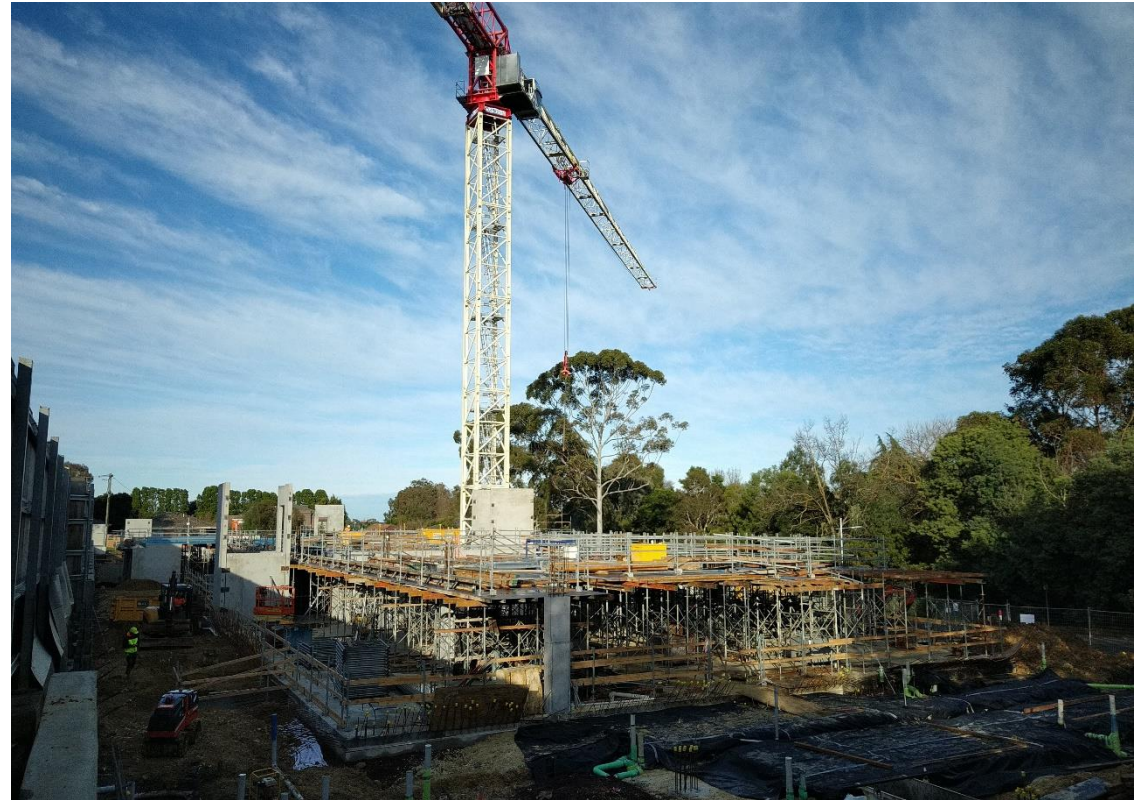
Development progress (July 2023)
